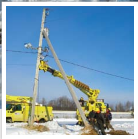
Cloverland lineworkers (L-R) Dan Brady, John Paquette Jr., and Jared Kangas use an auger to dig through layers of frozen ground at the I-500 Track in Sault Ste. Marie.
