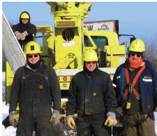
Edison Sault Electric lineworkers (L-R) Don Press, John Paquette Sr., Roger Bawks and Jeff Benoit (back) help relocate utility poles during an I-500 weekend workbee.
