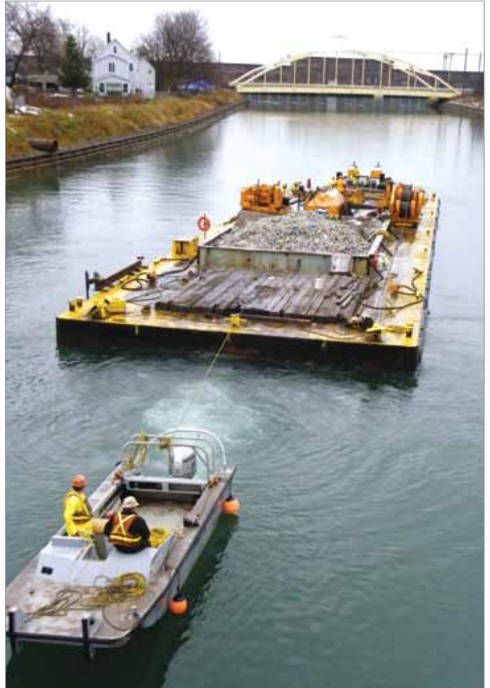
Final Voyage – A work boat helps guide the barge through the hydro canal to its winter storage dock next to the hydro plant. Canal maintenance finished for the season in late November.
