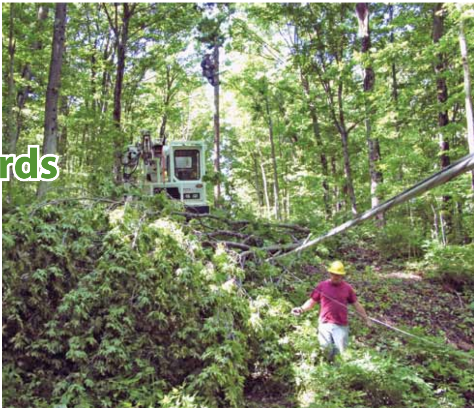
Great Lakes Energy crews rebuild a power line knocked down by trees during a summer storm last year.
