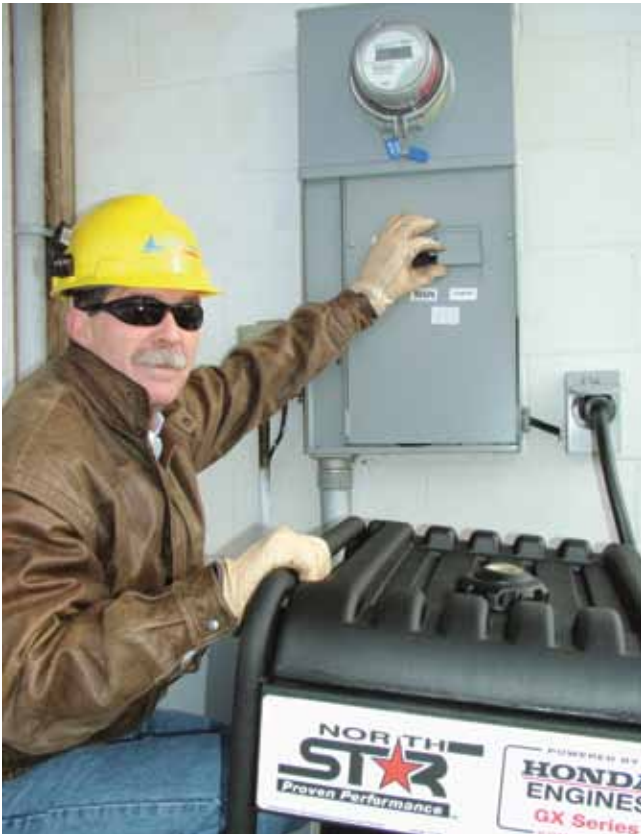
Dave Matz, Great Lakes Energy's operations director, points out the safety transfer switch that allows a portable generator to be safely connected to a home.
