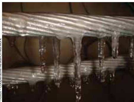
When freezing rain accumulates on electric lines, they become extremely heavy, often breaking and toppling support poles, which leads to power outages.
