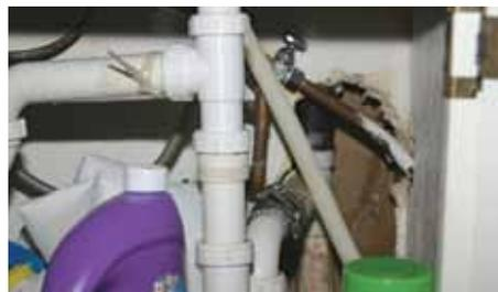
**Above:** Plugging open spaces around plumbing and other air leaks is an easy fix that saves energy and money.
