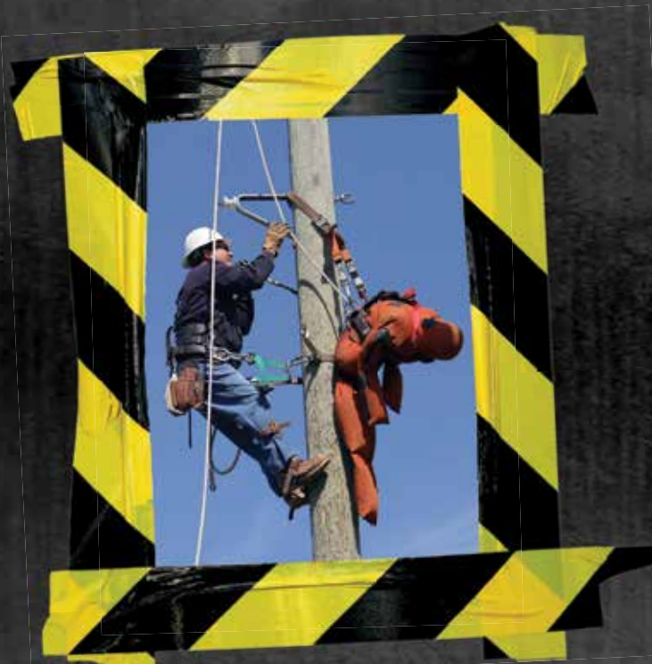
HomeWorks lineman Adam Doughty works through a recent pole top and bucket rescue training exercise.
