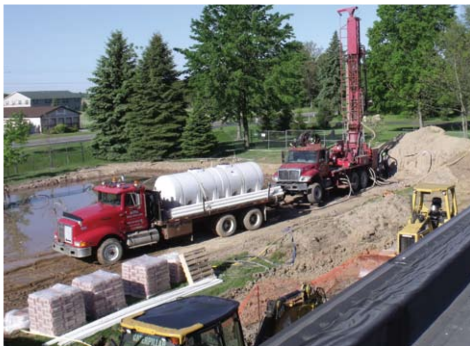
This photo, taken in mid-May from the roof of the former generator building by purchasing agent Deb Rogers, shows well drillers hard at work putting in new wells for the geothermal heating and cooling system at the cooperative's Portland office. Construction is on-schedule and the customer service lobby should re-open in August.
