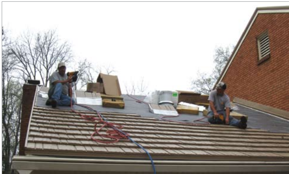
The metal roofing panels are installed over the underlayment. Hidden stainless steel nails and aluminum clips are used to secure each panel.
