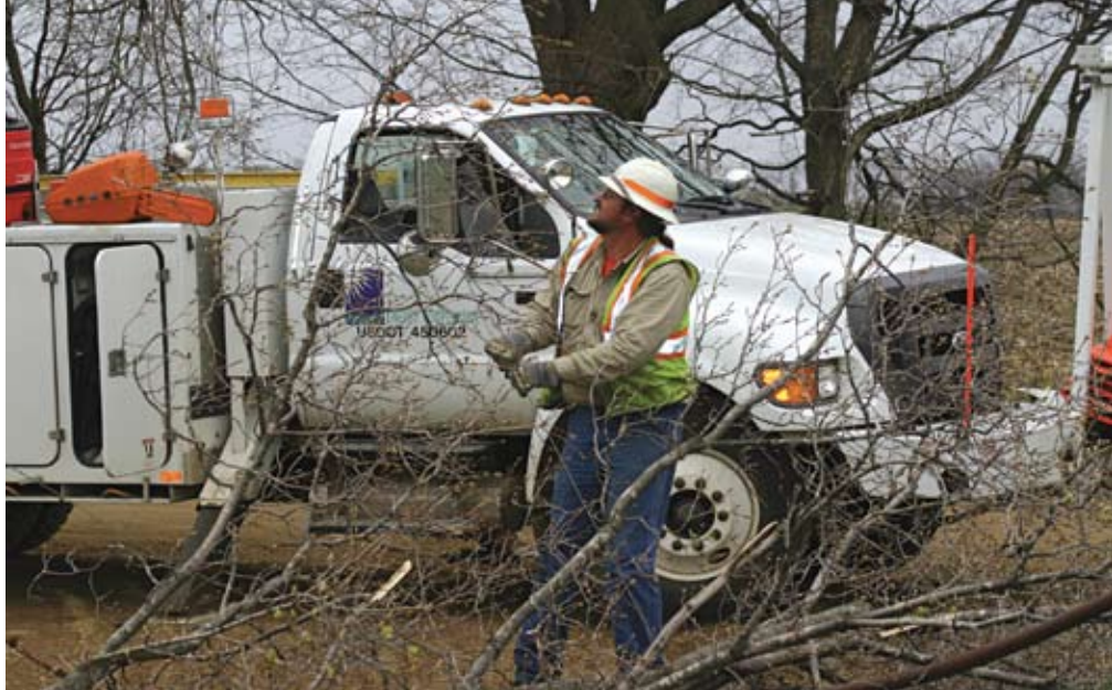
Midwest Energy Lineman Steve Stange tries to pull wire through a mess of downed branches during outage restoration. Below: High winds broke and scattered utility poles across the landscape and caused extensive damage to buildings.
