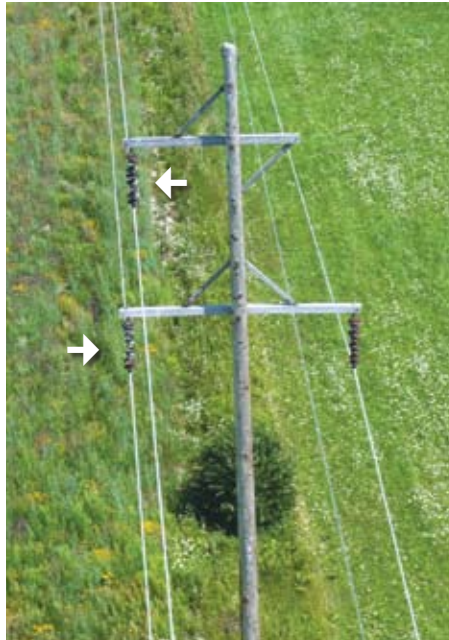
Damage to porcelain insulators on Wolverine’s 138 kilovolt (kV) transmission line near Ludington was discovered during the August aerial patrol of the cooperative’s transmission system. The damage appeared to be caused by gunfire.
