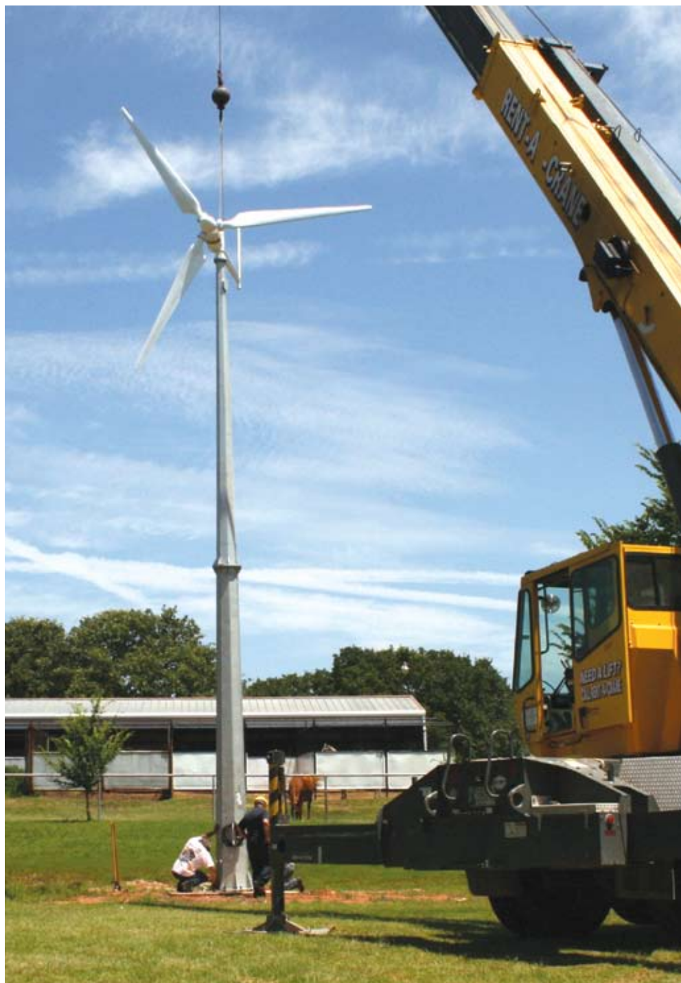
This small wind turbine stands about 46 feet tall, compared to the 300 feet reached by utility-scale wind turbines.
