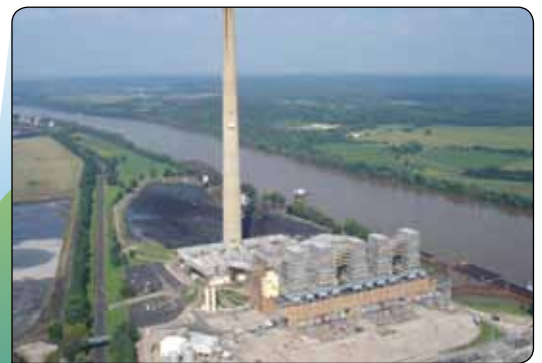
Located near Gallipolis, OH, the Kyger Creek plant has five 217-megawatt units.
