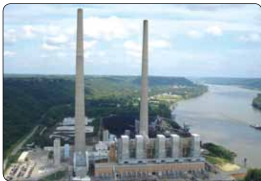
The Clifty Creek plant is located in Madison, IN. It has six units capable of generating 217 megawatts each.
