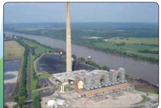
Located near Gallipolis, OH, the Kyger Creek plant has five 217-megawatt units.
