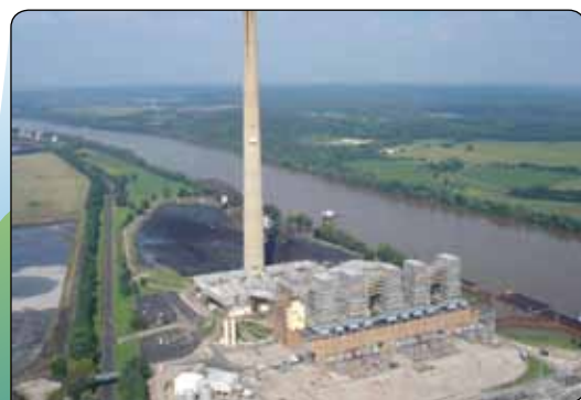
Located near Gallipolis, OH, the Kyger Creek plant has five 217-megawatt units.
