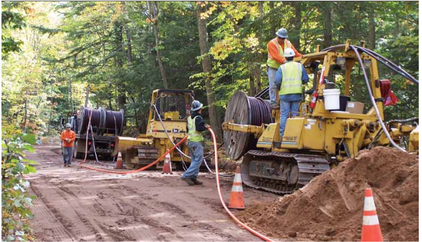
Construction crews prepare underground cables for installation to Kennecott Minerals.
