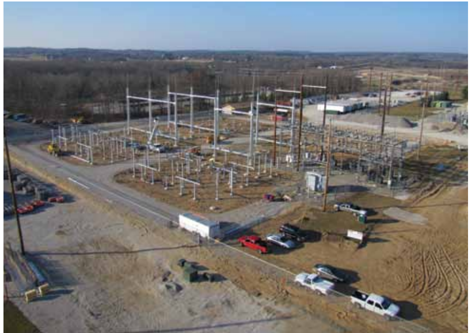
Wolverine Power Cooperative is constructing a new transmission substation near Hersey.
