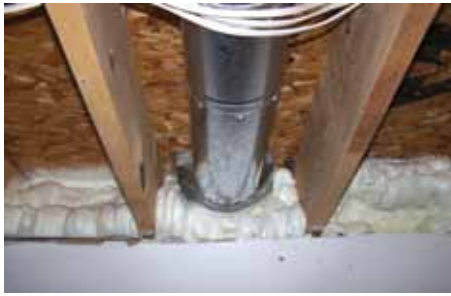
Spray foam insulation (applied by a contractor for large areas) can be used to plug air leaks and help you save money on your energy bill.
