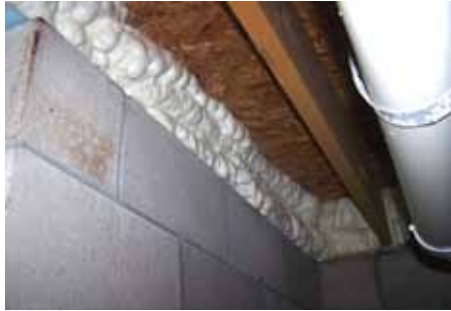
Spray foam insulation (applied by a contractor for large areas) can be used to plug air leaks and help you save money on your energy bill.
