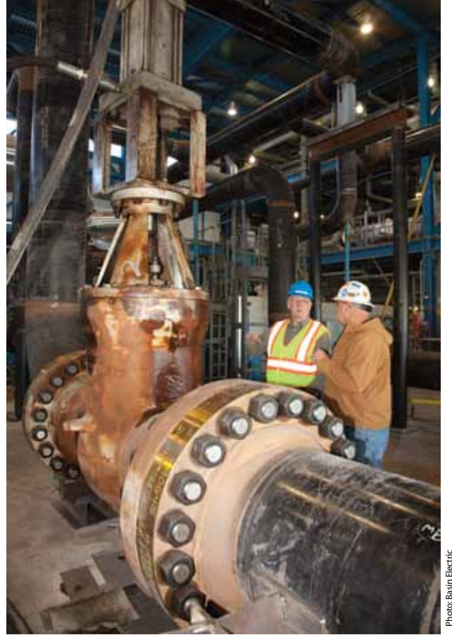
Photo: Basin Electric
