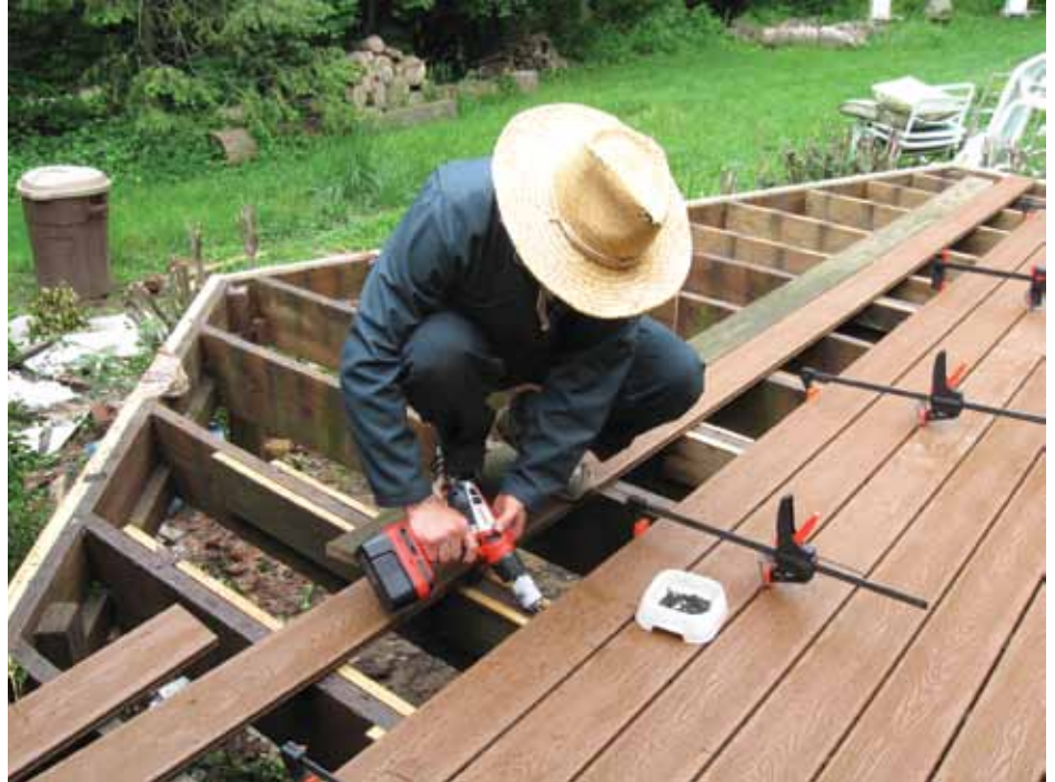
James Dulley is shown installing composite decking using hidden fasteners. Since these planks are not as rigid as wood, it is important to make sure you have proper maximum spacing between the joists.
