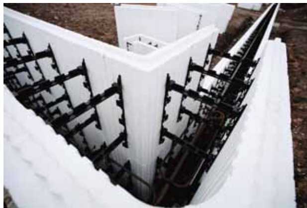
These insulated concrete forms use webs between the foam side to create the width of the gap for the concrete.
