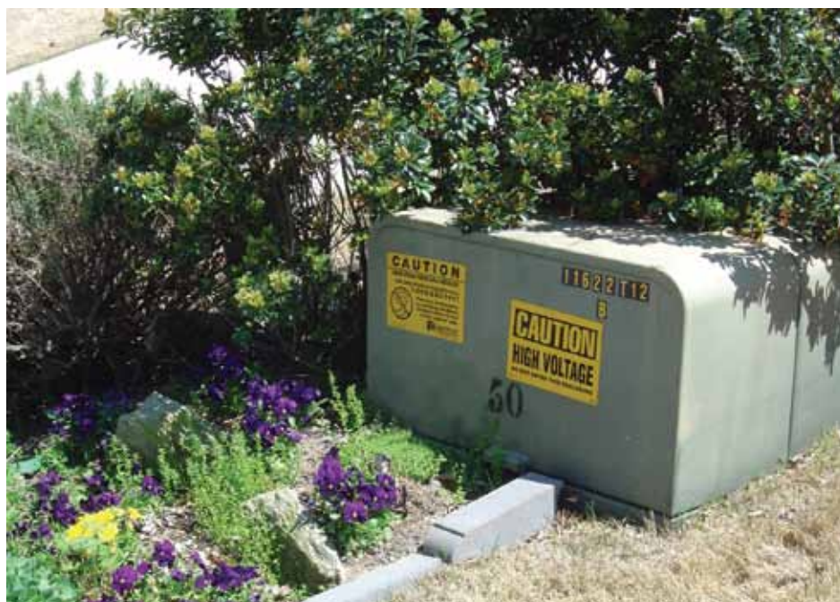
Never let anything grow closer than 10 feet from the access panel of your home's pad-mount transformer. How do you know where the access panel is located? Look for the handle, lock, and sticker. This distance keeps roots away and air flowing around your home's unit.
