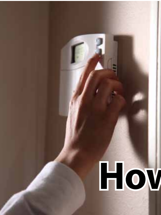
Source: Touchstone Energy
