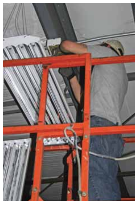
An electrician from Midwest Energy Group installs new lighting at Postle Extrusion through our Energy Optimization Commercial and Industrial Program.
