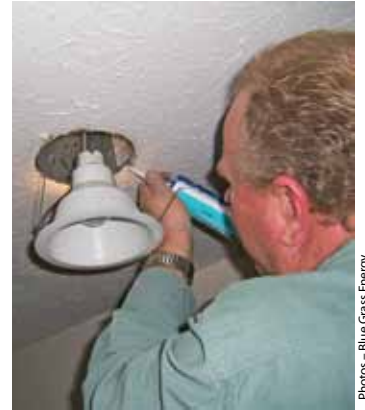
Black marks on your insulation (L) means there is air infiltration, and your insulation is doing little more than catching dust. Create an air barrier for more comfort and lower energy bills. Sealing the cracks around recessed can lights (R) with caulk can greatly reduce air flow.
