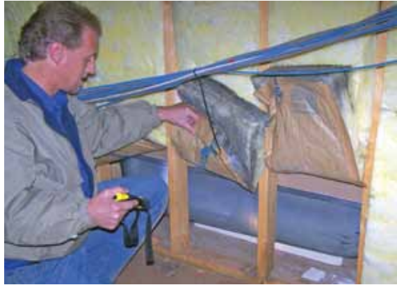
Black marks on your insulation (L) means there is air infiltration, and your insulation is doing little more than catching dust. Create an air barrier for more comfort and lower energy bills. Sealing the cracks around recessed can lights (R) with caulk can greatly reduce air flow.
