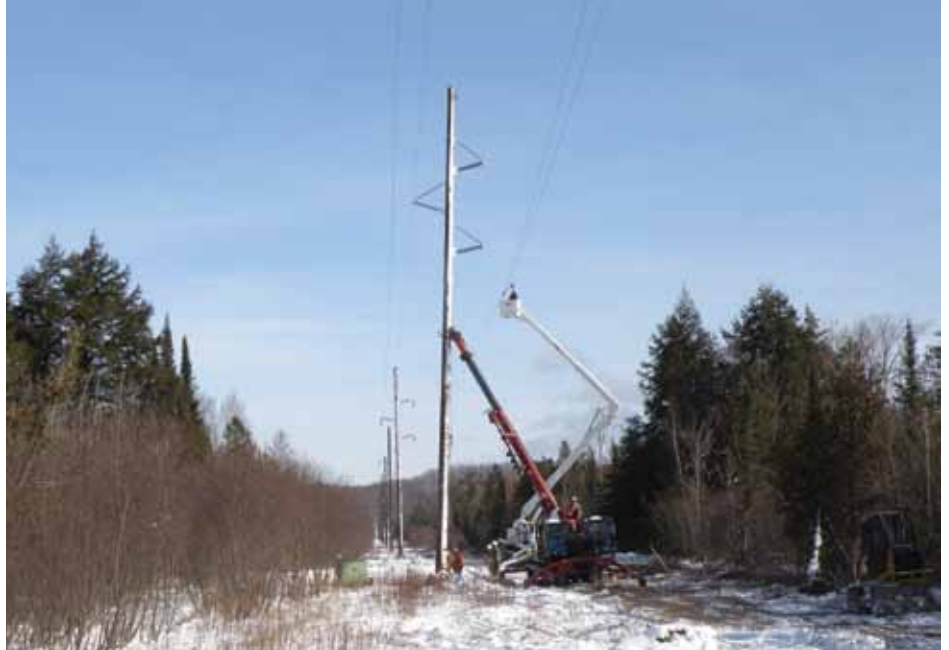
Wolverine lineworkers upgraded a section of the transmission system between Petoskey and Boyne City in February 2011 by installing new poles and wire.
