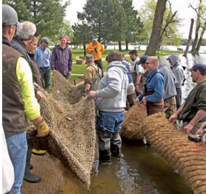
During the field component of training for becoming a Certified National Shoreline Professional, participants lay erosion control fabric and set coir fiber logs as wave breaks to protect the newly-constructed natural shoreline at Cadillac Lakefront Park.
