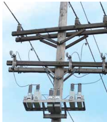
Capacitors improve the power on the lines—they prevent it from being wasted and help boost the voltage on long distribution lines.
