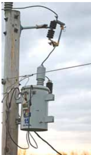
Transformers lower voltage to a level that's safe for use in your home.
