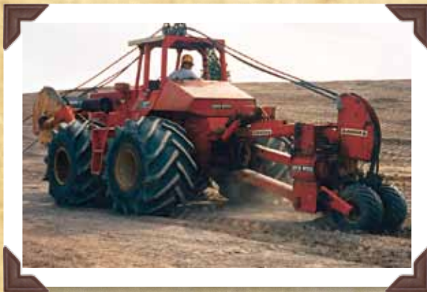
Underground cable being buried by a lineman using a Ditch Witch R-200. Just one of the machines used for underground installation.
