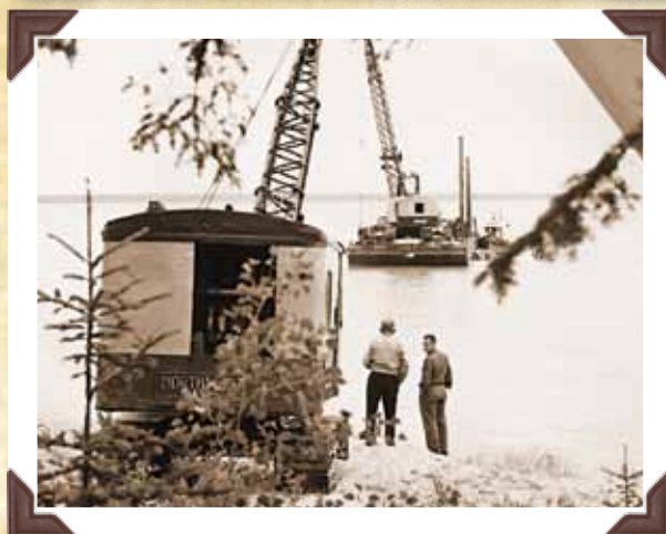
In the photos above, the surveyor is helping keep the cable on course with the help of Harry Pauly (in truck 51) relaying directions via truck radio to the barge across the 3.7 miles from Point Nipigon to Bois Blanc Island.
