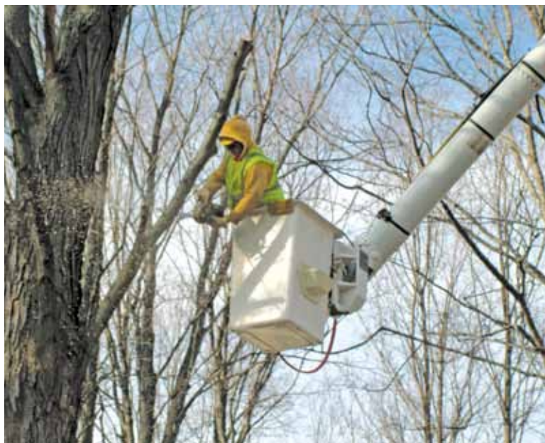
Photo – Great Lakes Energy
