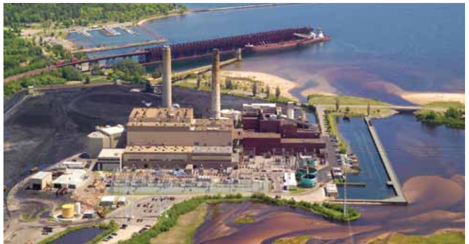
We Energies' Marquette power plant.
