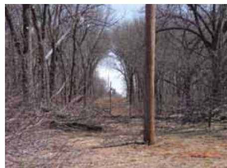
▼ The ground-to-sky approach to line clearance helps to make sure that trees don't form a canopy over the lines.
