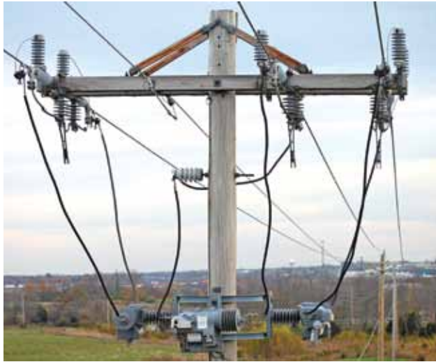
Reclosers protect lines and consumers from short circuits and allow temporary faults to clear, which helps keep service energized without needless interruptions.
