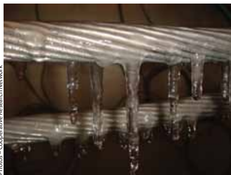
When freezing rain accumulates on electric lines, they become extremely heavy, often breaking and toppling support poles, which leads to power outages.
