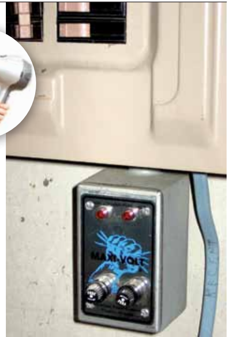
This whole-house surge suppressor mounts on the circuit breaker panel inside your home.
