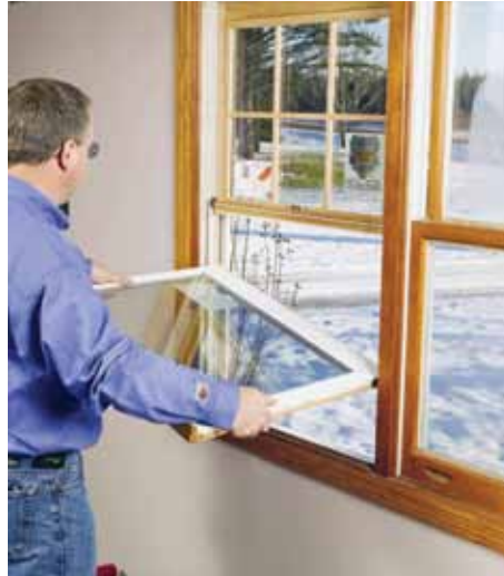
Tilt-in, double-pane, sash-only replacement kits provide a convenient way to convert old windows into efficient ones, if your existing frames are in good condition.
