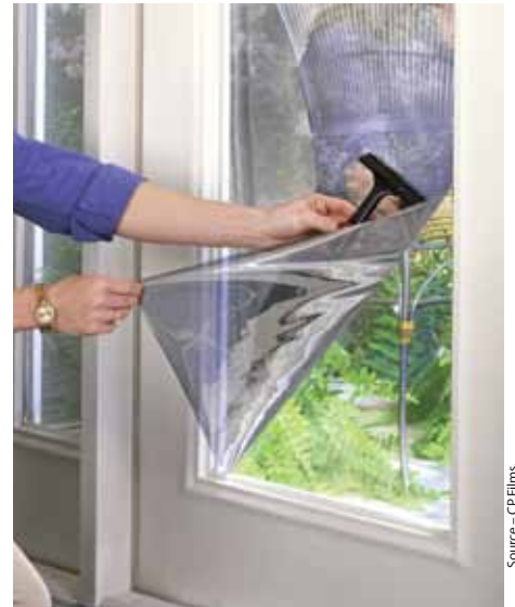
Energy-saving window film is installed on clean, wet glass using a squeegee to eliminate bubbles.
