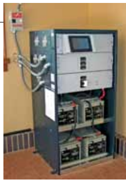
Home battery backup units (shown without a cover) are about the size of a refrigerator and generally fit in basements or spare rooms.
