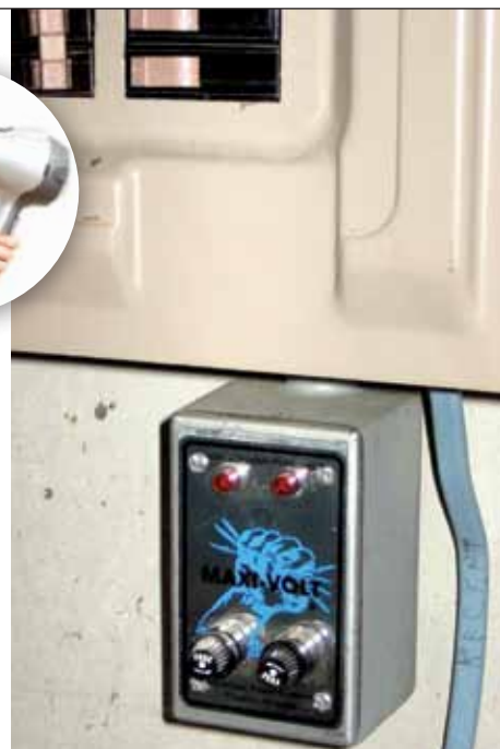
This whole-house surge suppressor mounts on the circuit breaker panel inside your home.
