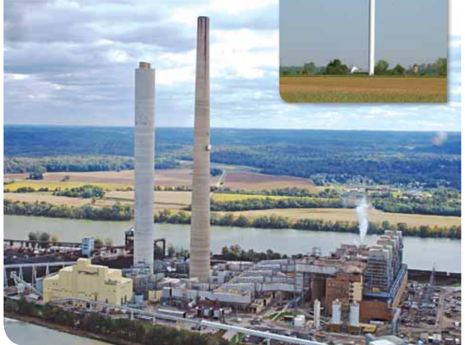
Kyger Creek Plant and Harvest Wind Farm, inset.
