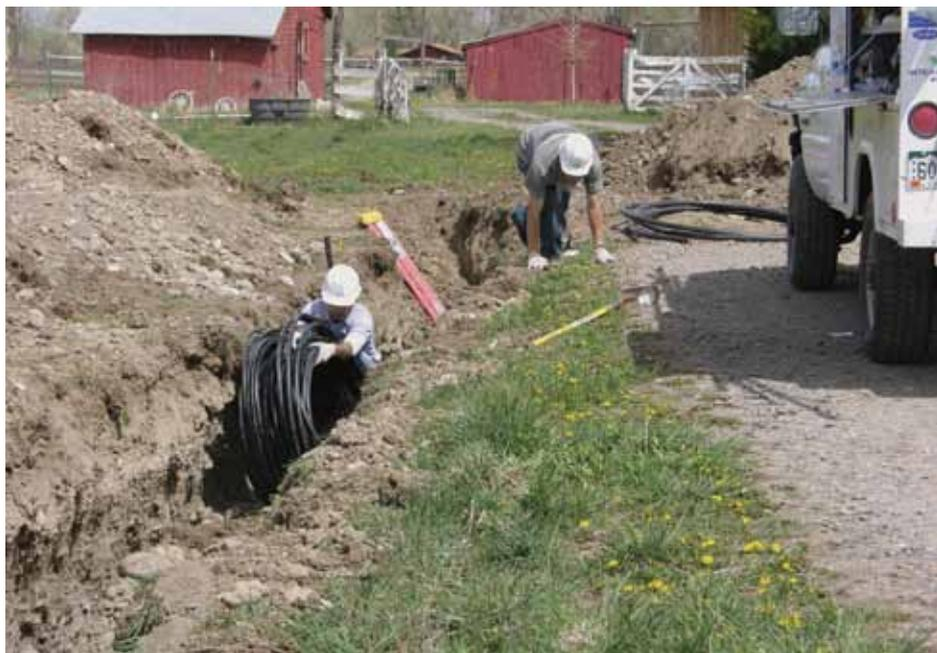
A knowledgeable and trustworthy contractor is a must when choosing a new heating and cooling system because he or she will install and maintain your unit for many years. Here, contractors install a geothermal heat pump "loop" system.
