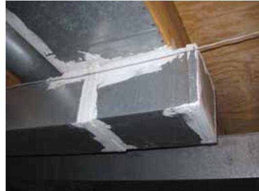
Seal seams in the ductwork where there are visible gaps or you can feel heated or cooled air leakage.
