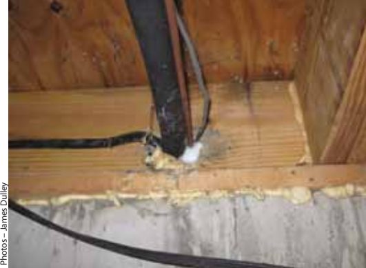
Check for gaps and air leaks where the sill plate rests on the top of the foundation.
