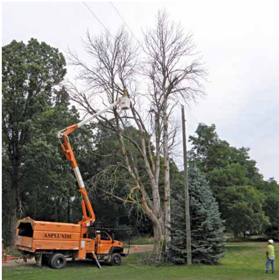
HomeWorks Tri-County contracts with Asplundh Tree Service to clear trees from our electric rights-of-way. Here, Joe Miller (in bucket) trims limbs from a dead ash before he and Rod Heikkila (on ground) take it down.
