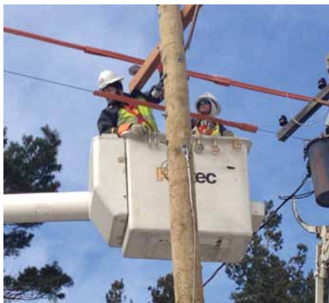
Lineworkers Jeremy Zbytowski and Kyle Balderson are shown connecting a newly-installed utility pole to the system (the old pole and transformer are shown at right.) Crew leader Chris Teachout directs from the ground.
