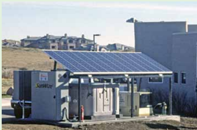
A combination of solar array and battery energy storage is another intriguing option that could help restore service to consumers more quickly by serving as limited power for a few hours. Paired with some type of distributed generation (such as a solar array), a battery backup, and enhancements to existing demand response systems (these offer incentives to consumers to reduce electricity use), limited power could potentially be extended to consumers indefinitely, even when the sun is not shining.
