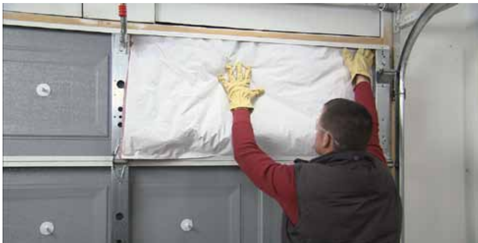
After clips are stuck to the garage door, fiberglass insulation batts are pressed over the clips.
