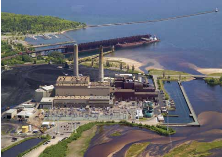
Aerial view of the Presque Isle Power Plant in Marquette.
