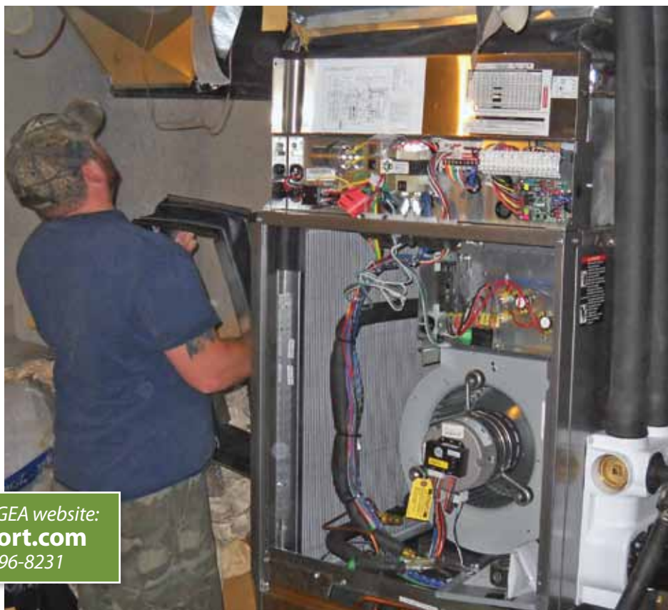
Installing the new geothermal unit in the Kaufman home in May 2013.
