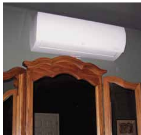
The indoor fan/coil unit is mounted high on the bedroom wall.
