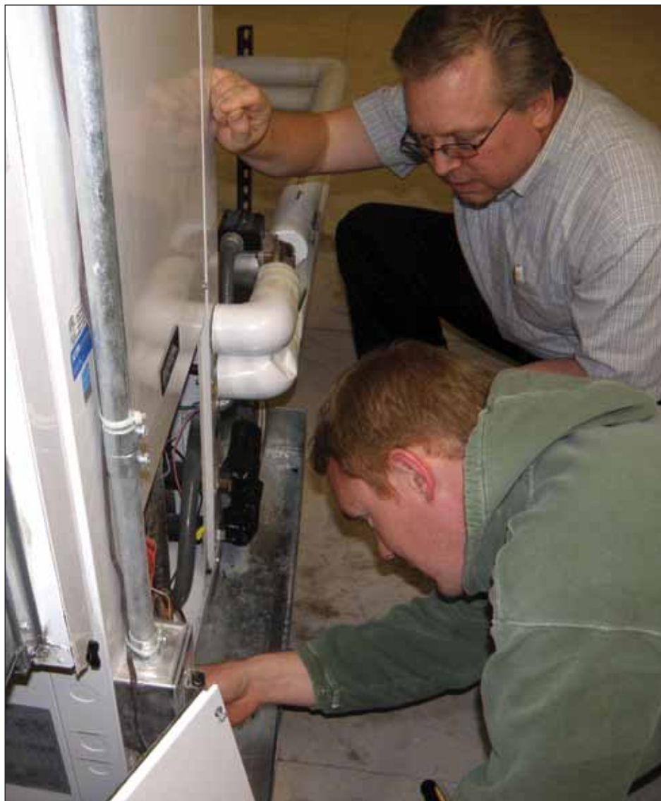
Tom Manting, top, and Nick Rusnell examine one of the geothermal units at HomeWorks Tri-County Electric's Portland office, setting them up for load management controls.
