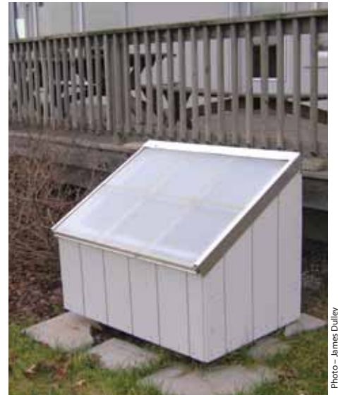
This do-it-yourself solar water heating kit uses a batch design to preheat incoming cold water.
