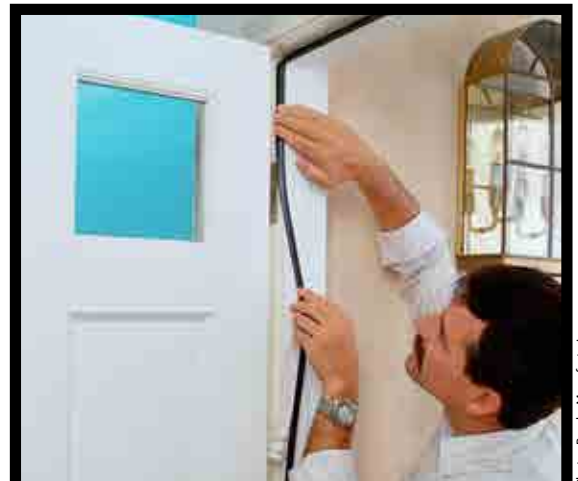
Replaceable vinyl weather stripping seals well on the door's hinge side because it gets compressed, with little rubbing and wear.
