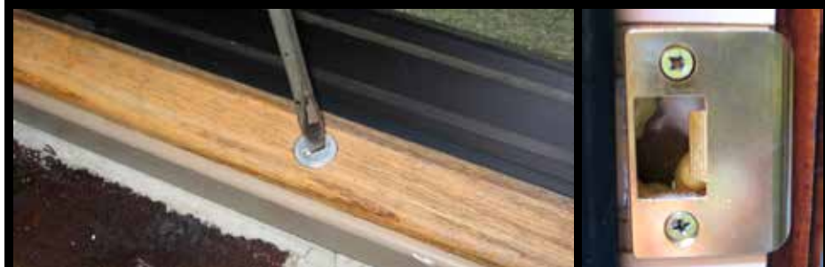
LEFT: A door's threshold can be raised or lowered with a screwdriver so the weather stripping seals tightly. RIGHT: Stepped teeth in this strike plate allow the door to fit tightly. Notice the small dab of expandable foam insulation inside.
