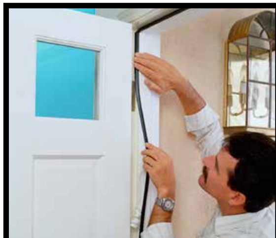
Replaceable vinyl weather stripping seals well on the door's hinge side because it gets compressed, with little rubbing and wear.
