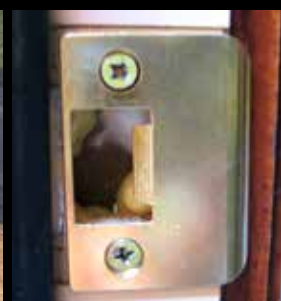
LEFT: A door's threshold can be raised or lowered with a screwdriver so the weather stripping seals tightly. RIGHT: Stepped teeth in this strike plate allow the door to fit tightly. Notice the small dab of expandable foam insulation inside.
