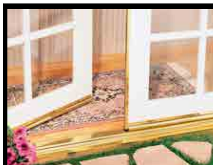
A new brass bottom seal and threshold save energy and are more attractive.
